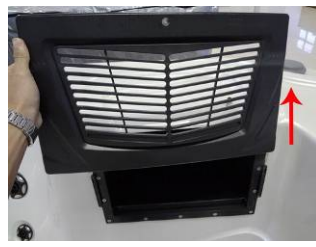
2. Take out the protection grating upwards.
